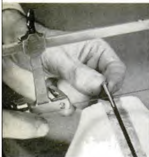
CHUNK OF BOLT can be whacked off (left) without leaving any burrs. Screw slot (right) that's clogged by paint or rust is quickly cleaned
